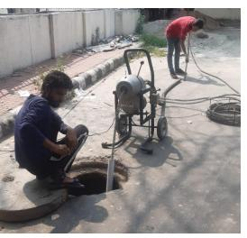
Our KAMBORE is a Motorised Outdoor drain cleaner for 4" to 12" lines which performs high speed drilling along with force and is the most effective way of removing blockages, be it in Mumbai, Bangalore or Delhi.
